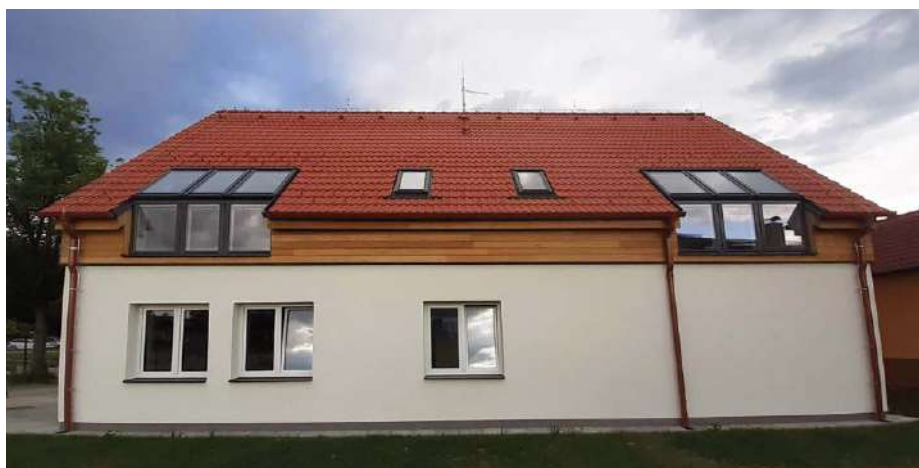
Photograph of the building.
