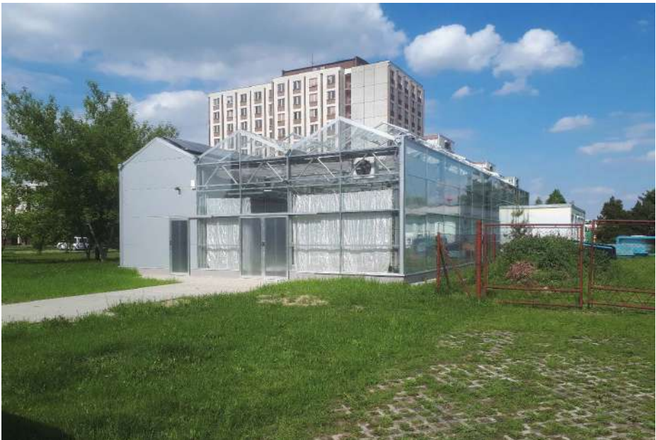
A newly built research aquaponic hall on the university campus.
